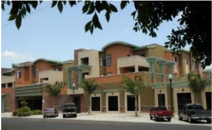
Colonial House Apartments, Oxnard
